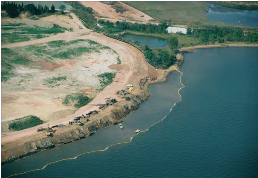
Photo A. Turbidity control with containment fencing
