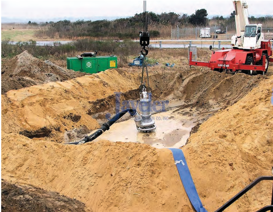
Photo A. Pit for slurry mixing (dry to wet material) and slurry pump
