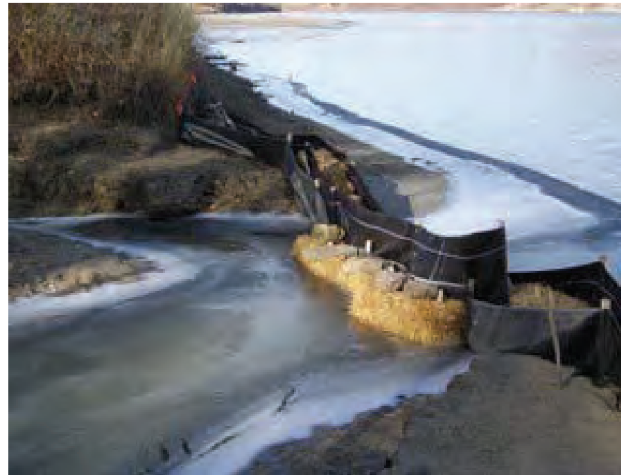
Photo B. Turbidity control with containment fencing www.terraerosion.com
