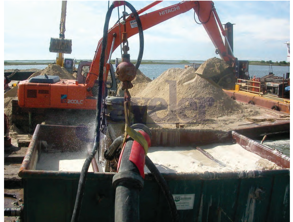
Photo B. Dump box for slurry mixing (dry to wet material) and slurry pump
