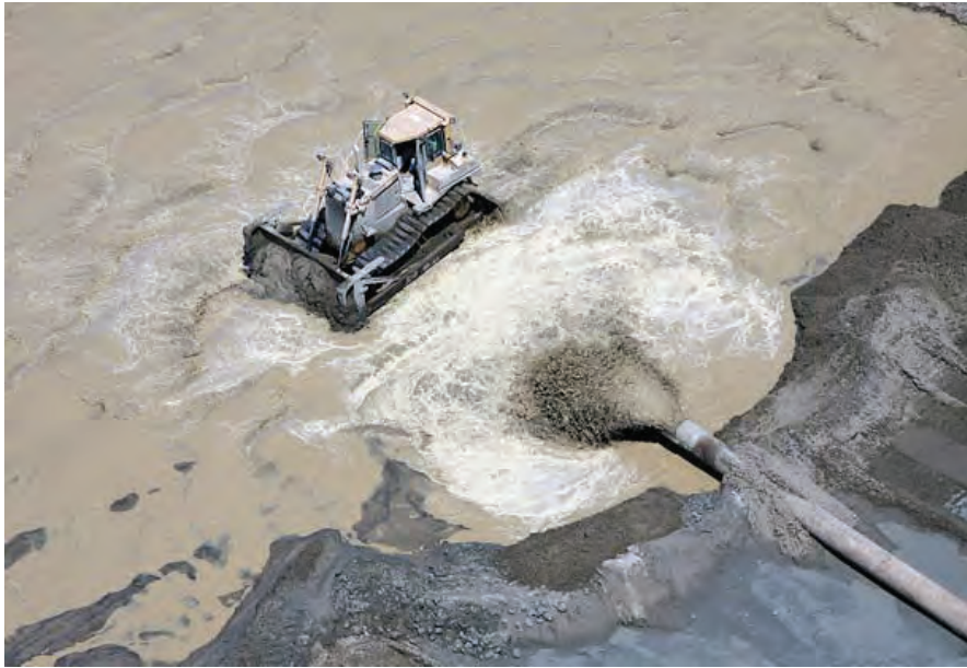
Photo A. Bulldozer clearing pipe discharge http://baynature.org/
