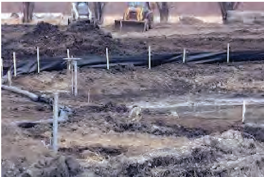
Photo C. Silt Fencing around a channel
