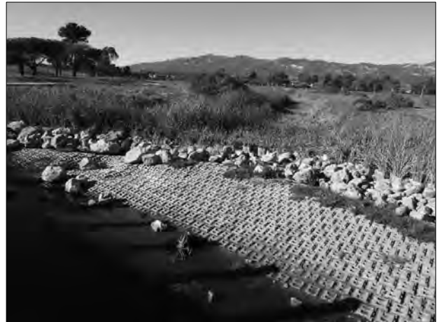
Photo 20: View north at Devereux Creek sheet pile sill separation from Devereux Slough tidal influence. 11/20/2015
