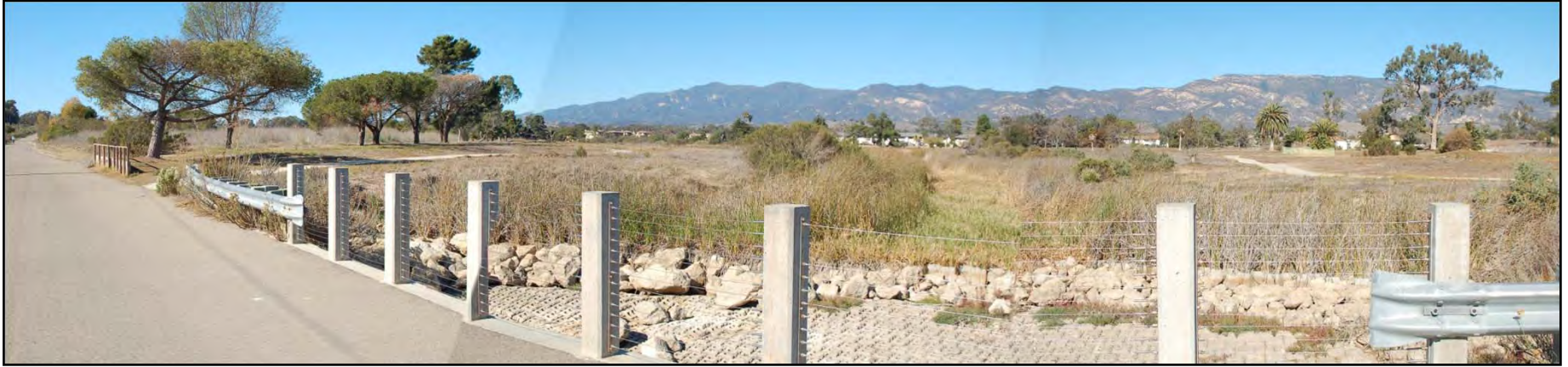
6. View from the Venoco Road bridge looking north across the South Parcel. Rip rap and bank armoring for the bridge can be seen in the foreground.
