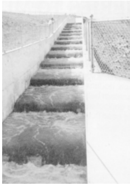
PHOTO: BUREAU OF RECLAMATION
