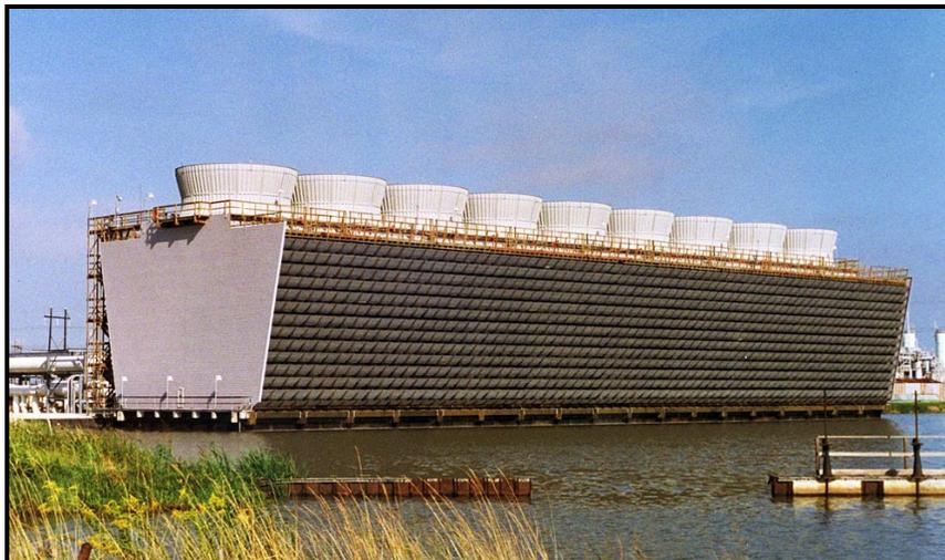
Figure 4–2. Multi-cell Mechanical Draft Cooling Tower
