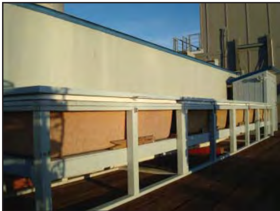
Live Fish Holding Tanks, MBCFO Wharf
