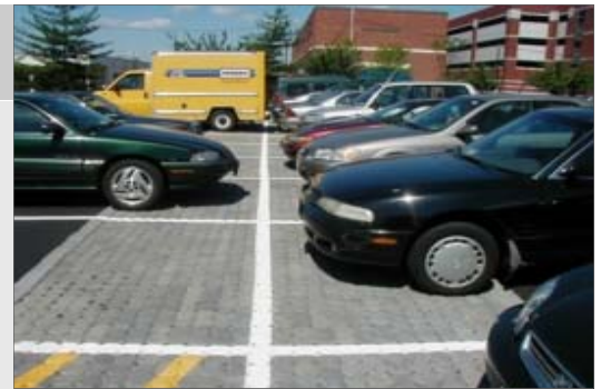
Porous pavement covers about 1/3 of each parking space in the D.C. Navy Yard parking
