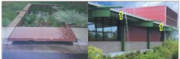
Stormdrain leading to bioretention cell
