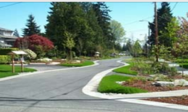
LID street design: vegetated swales, no curbs, and narrower streets promote infiltration of stormwater.
